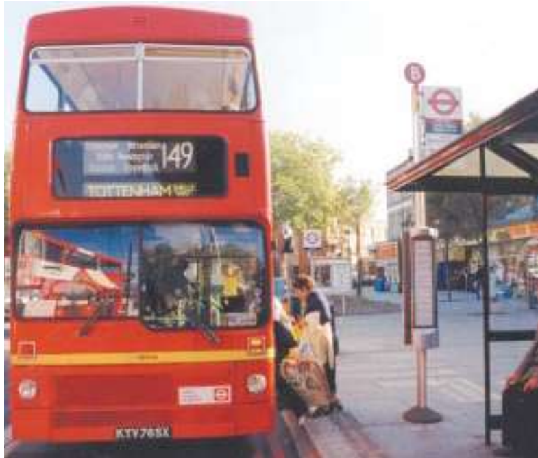
Footway and bus stop improvements have been made at the Seven Sisters interchange, London. Courtesy: TDFL.
