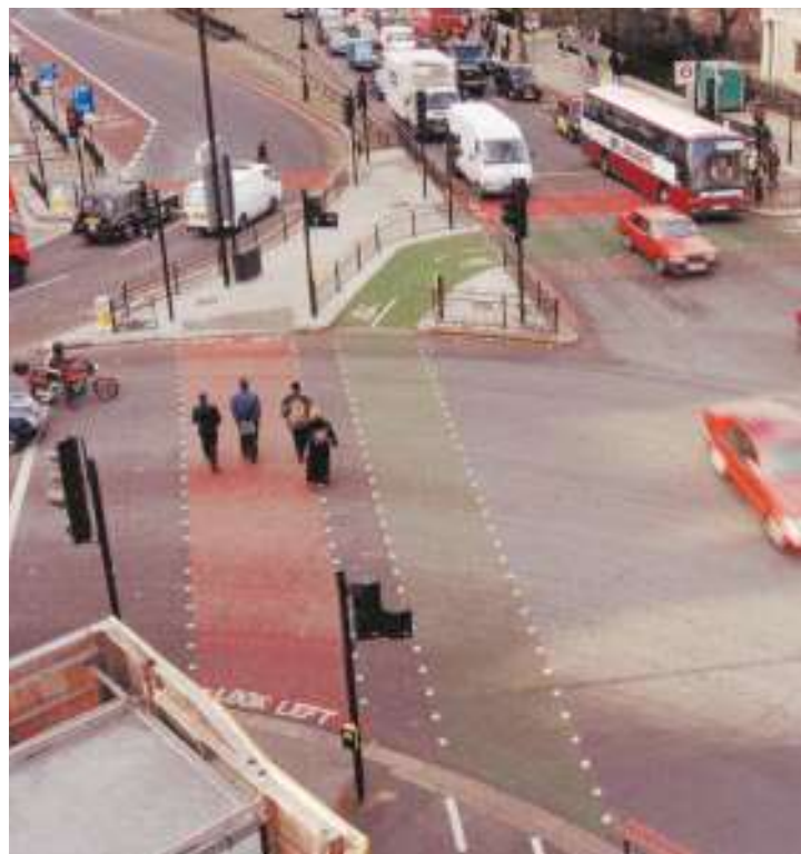
Hyde Park Corner – After: new at-grade crossing for pedestrians. Courtesy: TDFL.
